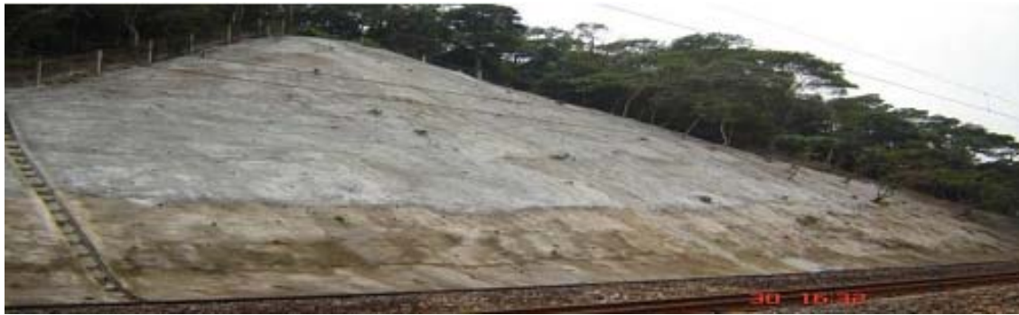
改善前 Before Improvement
